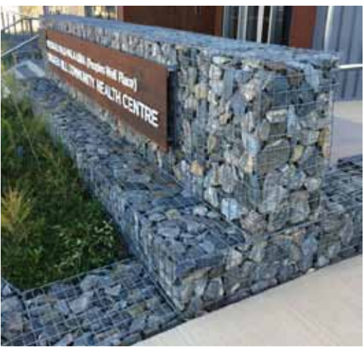
Low gabion wall
